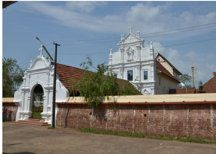
Fig 3, St Mary's Orthodox Church / Kottayam Cheriypalli, Kottayam, note the heavy wall and also the typical Portuguese entrance.
